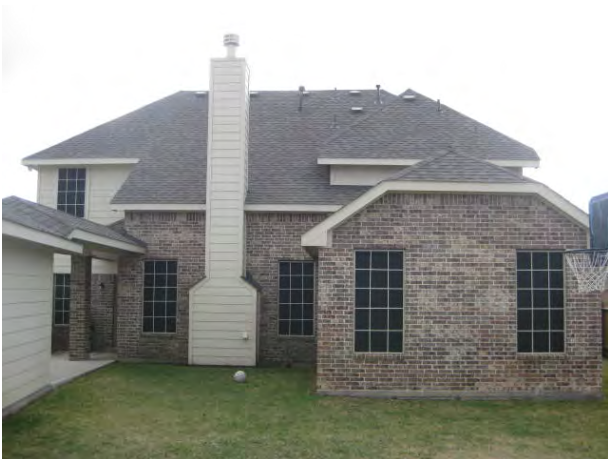
View: Back side of structure
