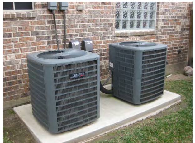
View: Back left side of structure at A/C
