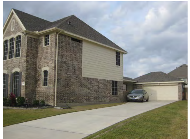
View: Front right side of structure
