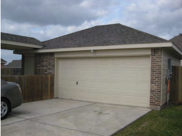
View: Front of detached garage
