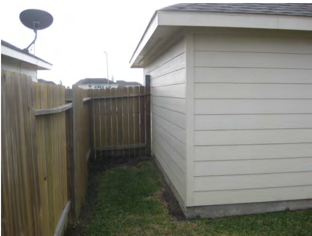
View: Back right side of detached garage
