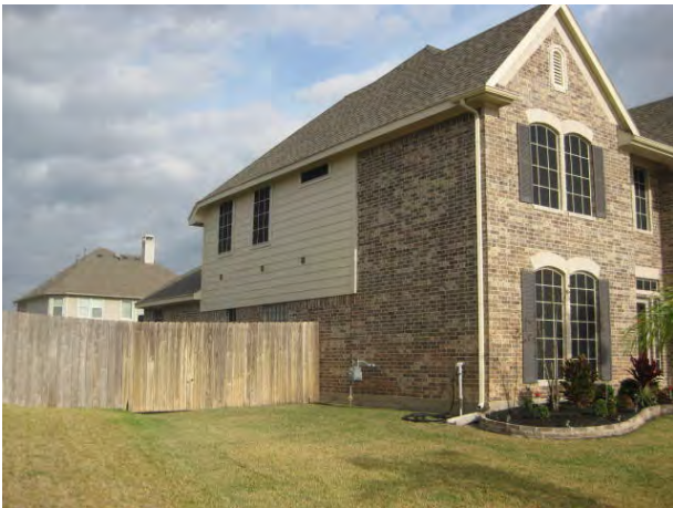
View: Front left side of structure
